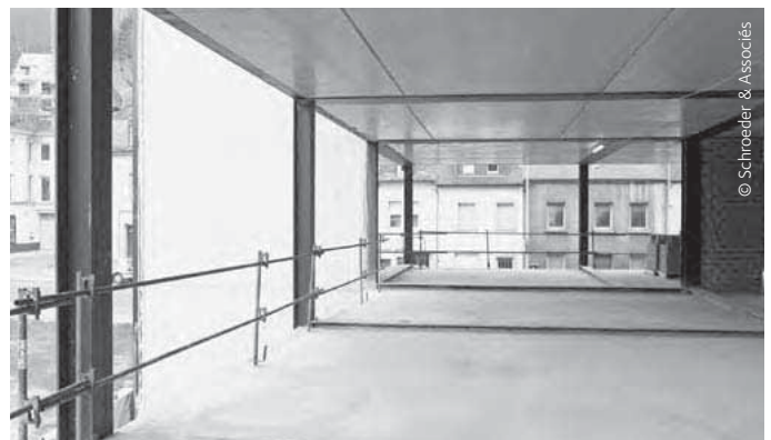
Figure 5.4.2 Underside of a finished floor
