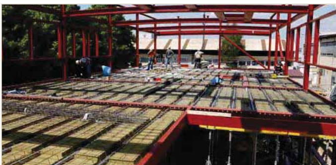
Figure 4.3 Examples of CoSFB. left: Maizières-lès-Metz (France). right: © atelier "Offermann" Mersch (Luxembourg).
