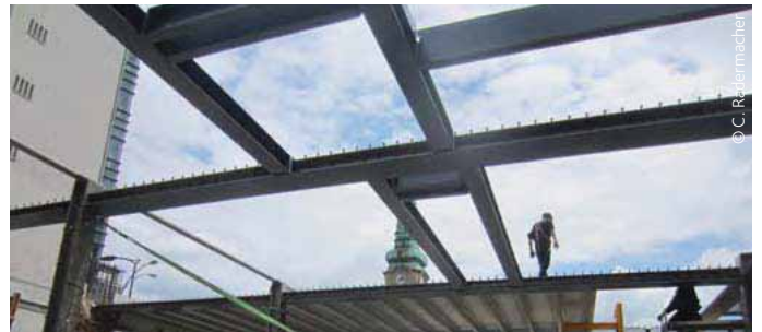
Figure 3.1 Galerie Kons (Luxembourg) – construction phase
