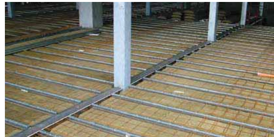
Figure 2.2 Slim-Floor beam application (Petrusse Building, Luxembourg)
