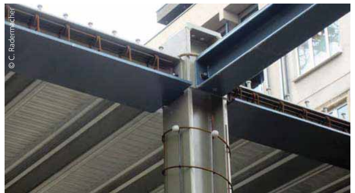
Figure 5.1 Beam-column joint
