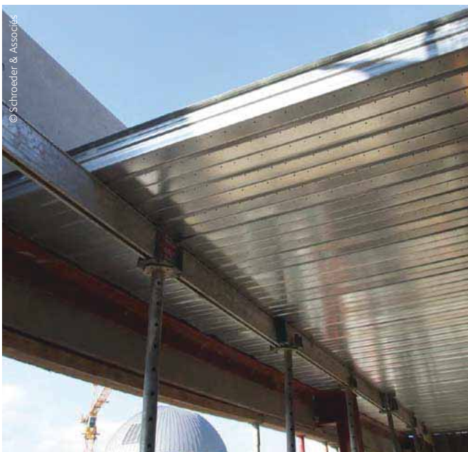
Figure 5.4.1 Temporary propping
