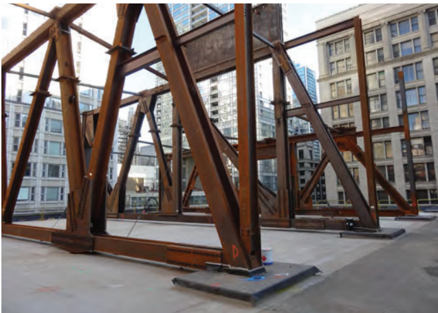
A913 Grade 65 sections used in transfer trusses
