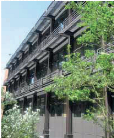
Office Building, Esch/Alzette (L)
